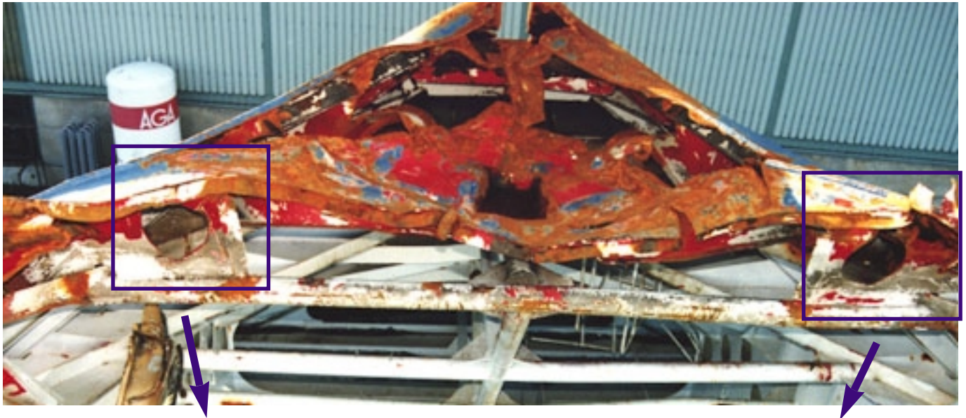
Picture 20. Overview of the bottom plate damage and details below.
